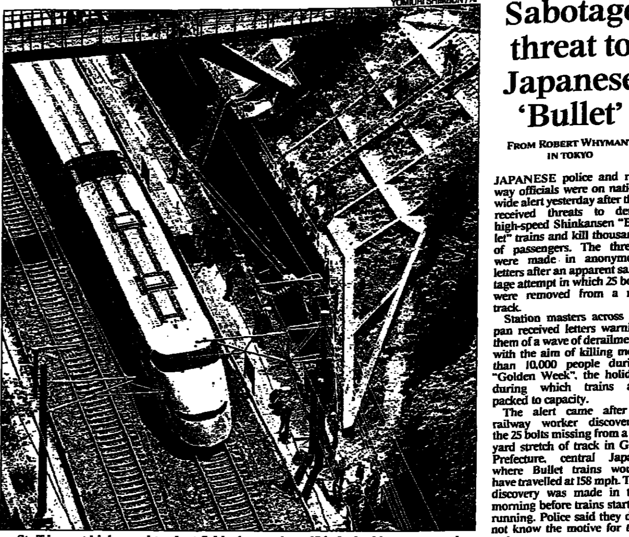
Staff inspect high-speed track at Sekigahara, where 25 bolts had been removed
